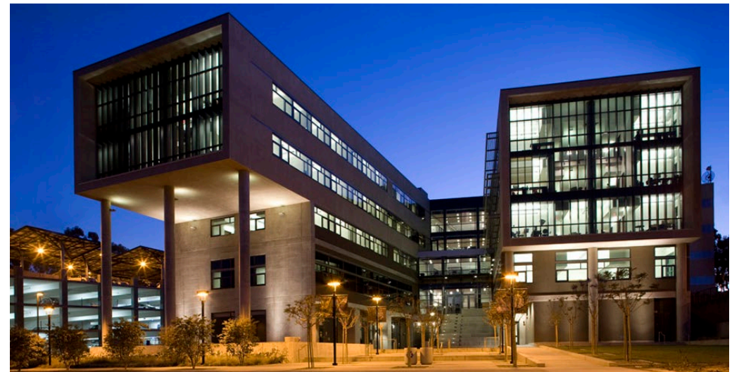
San Diego Supercomputer Center
